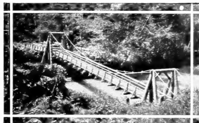
Thunder Creek suspension bridge
